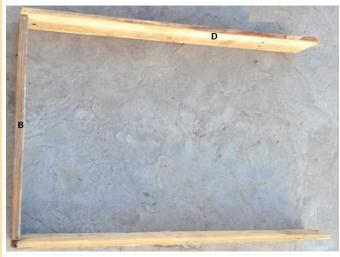
Let's build from the bottom to the top. Place one B piece between two D pieces. Then, nail it into place.
